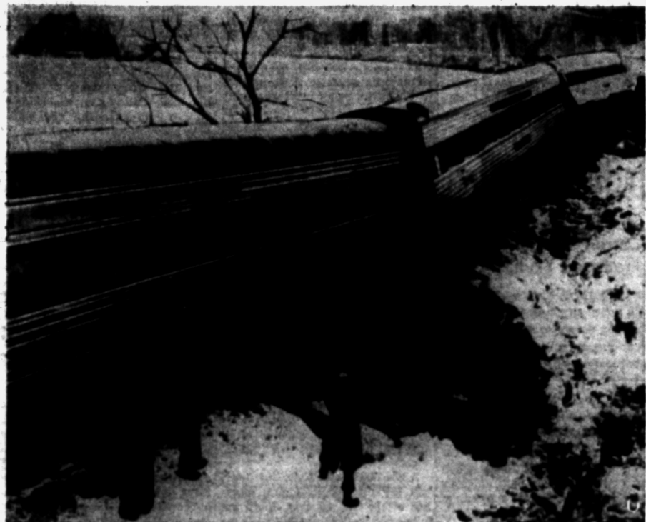
MAINE WRECK —The Maine Central passenger train "Pine Tree Limited" was wrecked by a washout near Augusta, Me. last night. Two milk cars in front of the train fell into the Kennebec River (background). No one was seriously injured, although three passengers were still in Augusta General Hospital early today. Doctors said they were listed as good.
