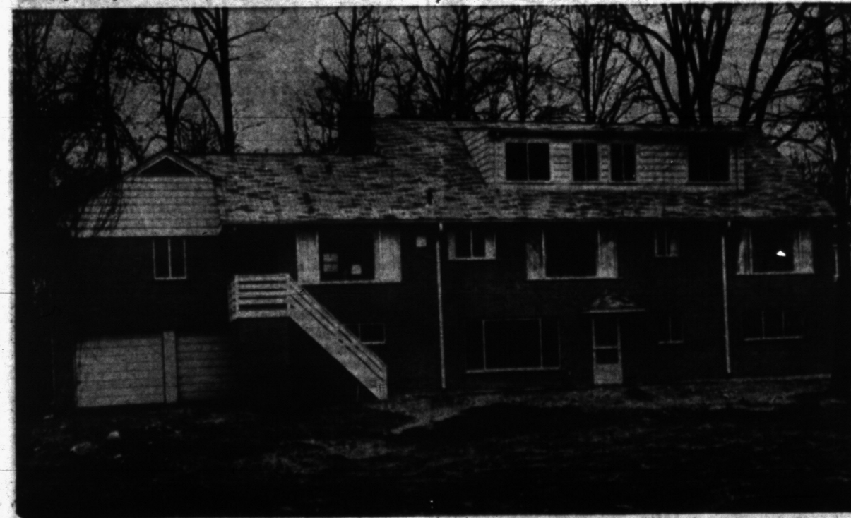
VIEW FROM LAKE REVEALS THREE FLOORS —Each of the three floors of the Annett home is a complete living unit of its own. First floor, only visible from the lakeside, has a large California redwood paneled recreation room, shower and powder room, laundry room, fruit and storage room and a garage space
