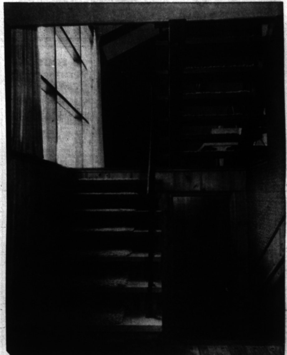
STAIRWAY TIES IN FOUR FLOORS —With a wrought iron railing and steps of pine planks, this four-level stairway makes all floors of this house accessible from a central spot. The lower floor is an activity room, laundry and furnace room. Second floor houses a family room, kitchen, bath, pantry and hallway. On the third floor is the formal living room, master bedroom, entrance hallway and bath. Children's sleeping quarters are three bedrooms on the fourth floor with a large full-tiled bath.
