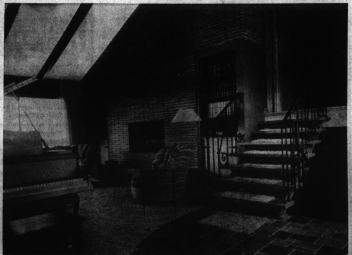
ROMAN BRICK FORMS ROOM WALL —The third-floor formal living room in the Geymans' house has one complete angled wall of Roman brick. A raised hearth fireplace centers this. The slanted ceiling has large wooden beams and the plastered ceiling
