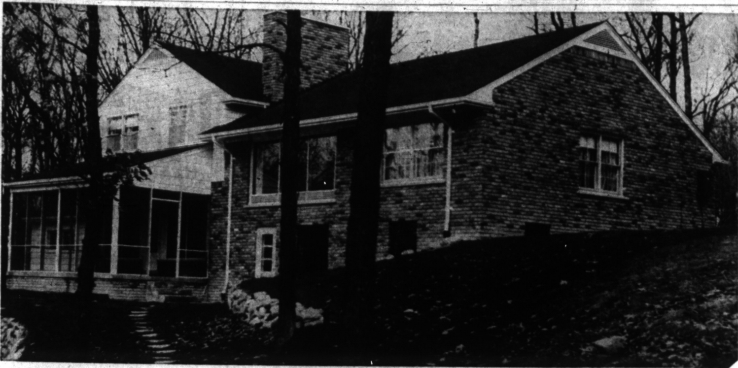
RECLAIMED BRICK EXTERIOR —Mellow color tones of reclaimed brick with sections of white clapboard provide an interesting exterior for the Jack Geymans' new home at 1465 Kirkway, back of Kirk of the Hills. An authentic split-level house, there are
