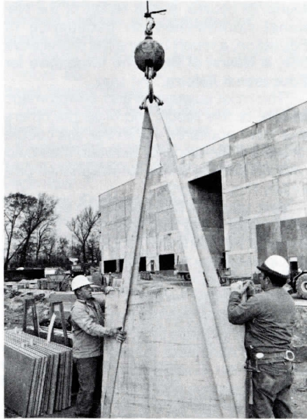
Construction is progressing at the Oakland Technology Park west of campus. Henry Lynch, left, and Charles Suder prepare a granite panel for the Comerica Bank building. Comerica is the high-tech park's first tenant.
