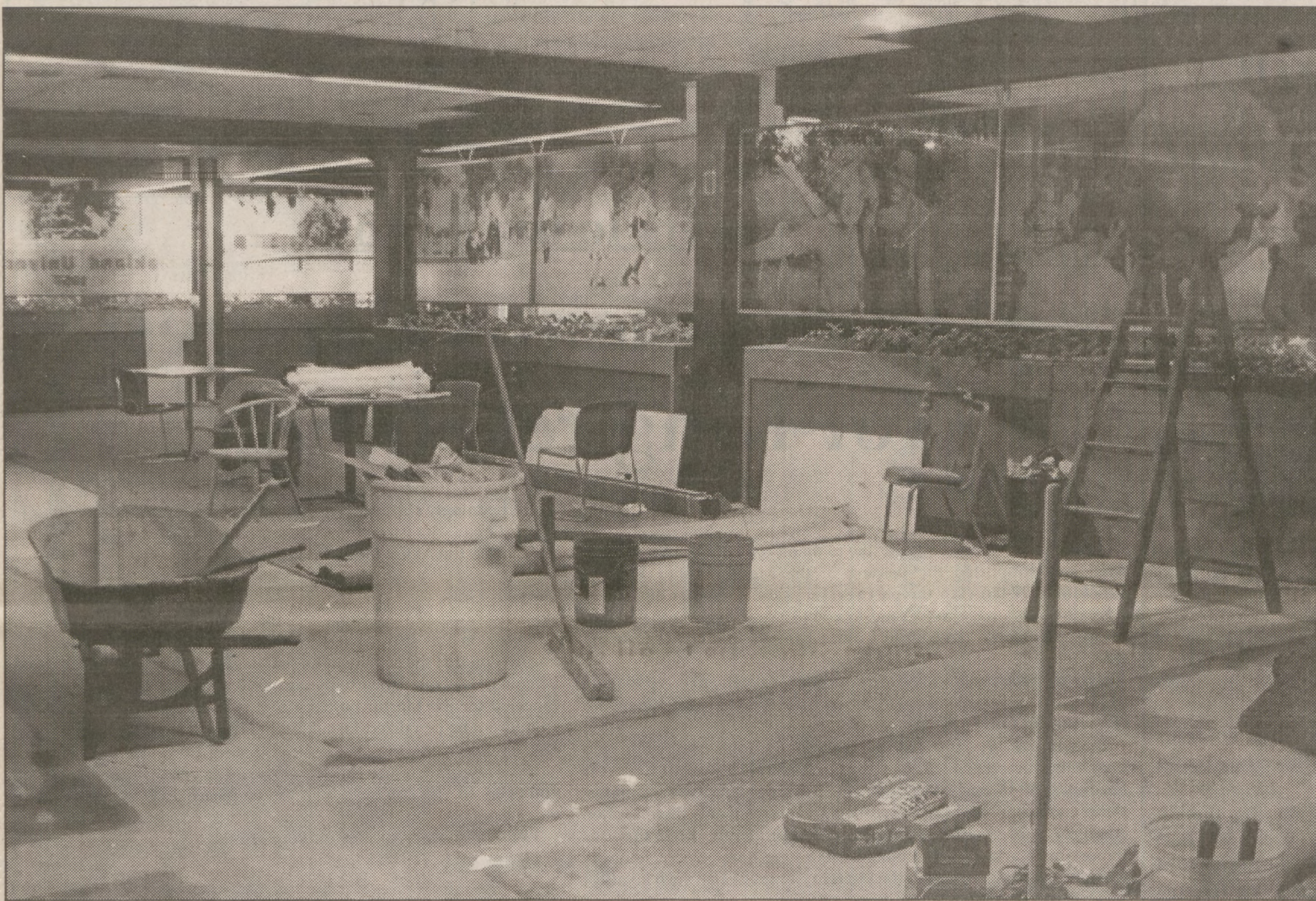
NEW LOOK: Richard Fekel, OC director, said the basement of the OC could receive a facelift in the future. Bids are currently being taken on the project.
