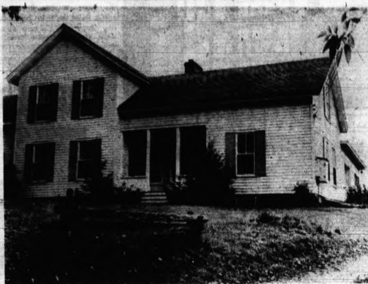
1950 EXTERIOR — Two wings, one at the left and one at the rear, have added space to this old farmhouse. Gone is the dark screened porch. The exterior is white with blue shutters. With all their remodeling behind them, the Toothachers can now settle down and enjoy country living.
