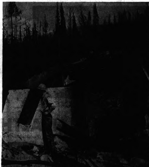
FIRE MELTS BRIDGE — The 2,000-degree heat of a forest fire near Sandpoint, Idaho, melted portions of this bridge including quarter-inch reinforced steel in the approach. Forester Gustav Verdal inspects the damage at Pack River Bridge yesterday in the Sundance Forest area.
