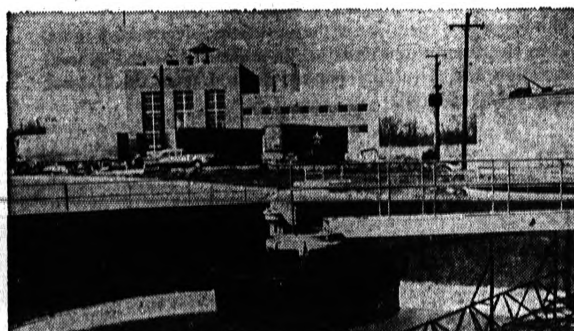
Completion of buildings and equipment for the new sewage treatment plant is expected early in 1963.
