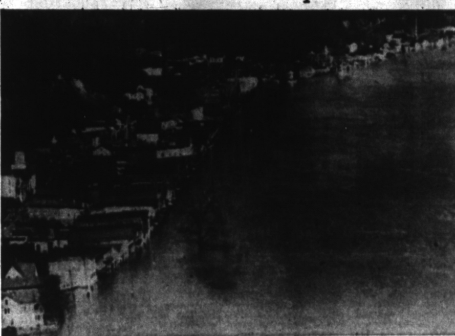
POMEROY SUFFERS DAMAGE — The business section of Pomeroy, Ohio, 200 miles east of Cincinnati, is shown inundated by muddy water from the flooding Ohio River. In the above picture the main business street is directly on the water and from bottom left to upper right is a distance of more than four miles.
