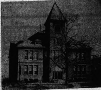
4. Central School on E. Pike Street (Pooled you on this one).
