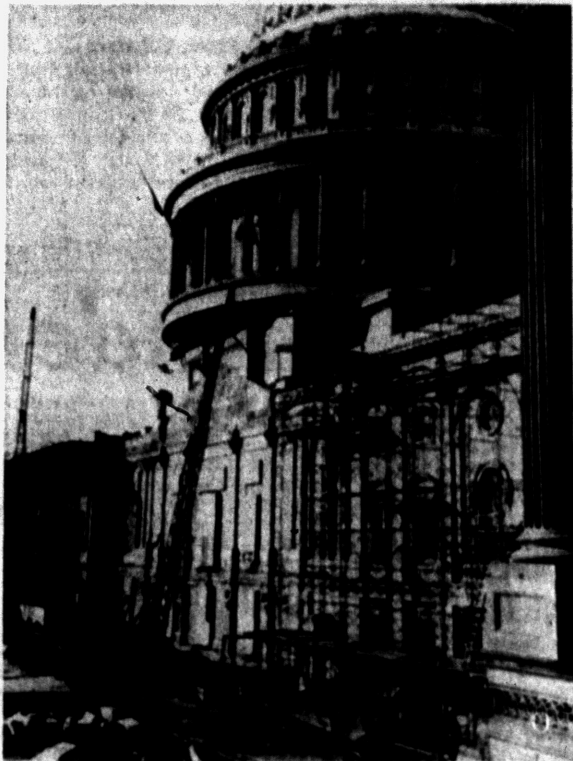
UNFAMILIAR LOOK — The United States Capitol — minus its wide center steps and massive pillars — presents this unfamiliar appearance as workmen continue the job of remodeling the structure. The view is from the Senate side of the building. The front will be extended some 30 feet and the steps and pillars replaced.
