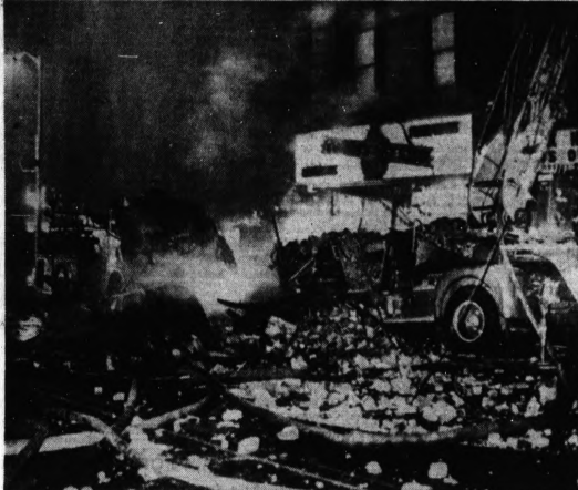
DEBRIS COVERS FIRE TRUCKS — Bricks and debris cover fire engines and hoses after a part of a wall collapsed during a fire at a Harlem Black Muslim Mosque in New York early this morning. Six persons were injured. One or more explosions were heard before the fire spread through the building.
