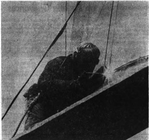
GETTING READY — Workmen throughout the city are preparing for the arrival of Detroit water in Pontiac. Tanks and other structures are being built, water lines being laid for the arrival of the water in early summer. (See story, photos on Page 17.)
