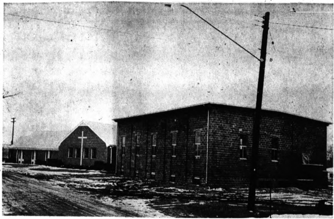
NEW ADDITION —The congregation of First Free Methodist Church is looking forward to the completion of the Christian Education Building being constructed adjacent to the present church. When finished it will house Sunday School classrooms and a Fellowship Hall for work and recreation.
