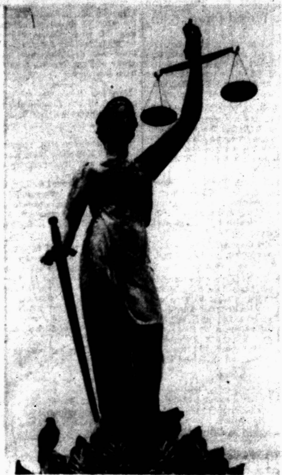
SCALES BACK — The Oakland County Courthouse tower is taking on a new look, as the dome is covered with aluminum paint. A workman (top picture) stands close to the figure of Justice as he hauls supplies from below to complete the regilding job. The scales of justice, missing from the lady's hand for a number of years, have been returned to their rightful place. Those birds in the extreme bottom of the lower picture are not part of the original architectural scheme, they just happened to be around when the picture was snapped.
