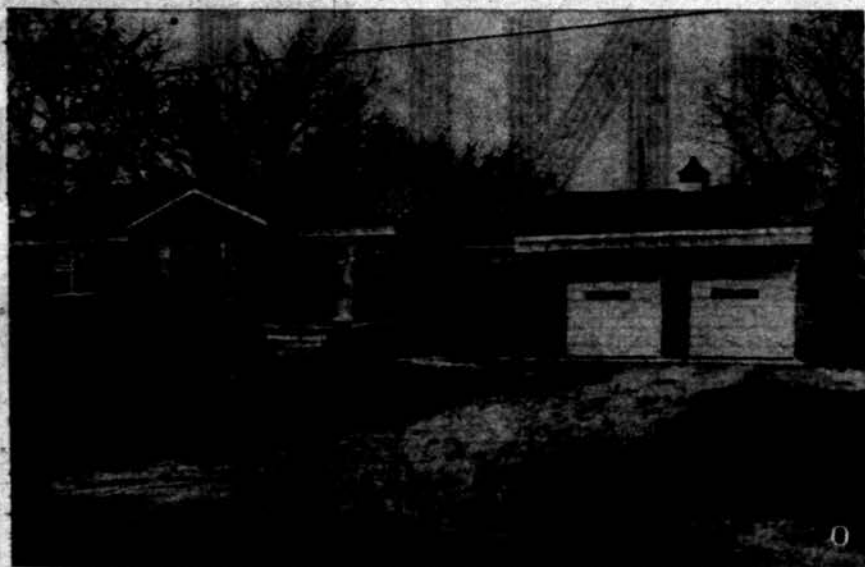
FAMILY PROJECT — This five-room house on Elizabeth Lake road was a family project for the C. M. Tarchalskis. While Mr. Tarchalski did most of the work, Mrs. Tarchalski helped in such ways as mixing mortar and sorting flooring. Even the children got in the act. Part of the
