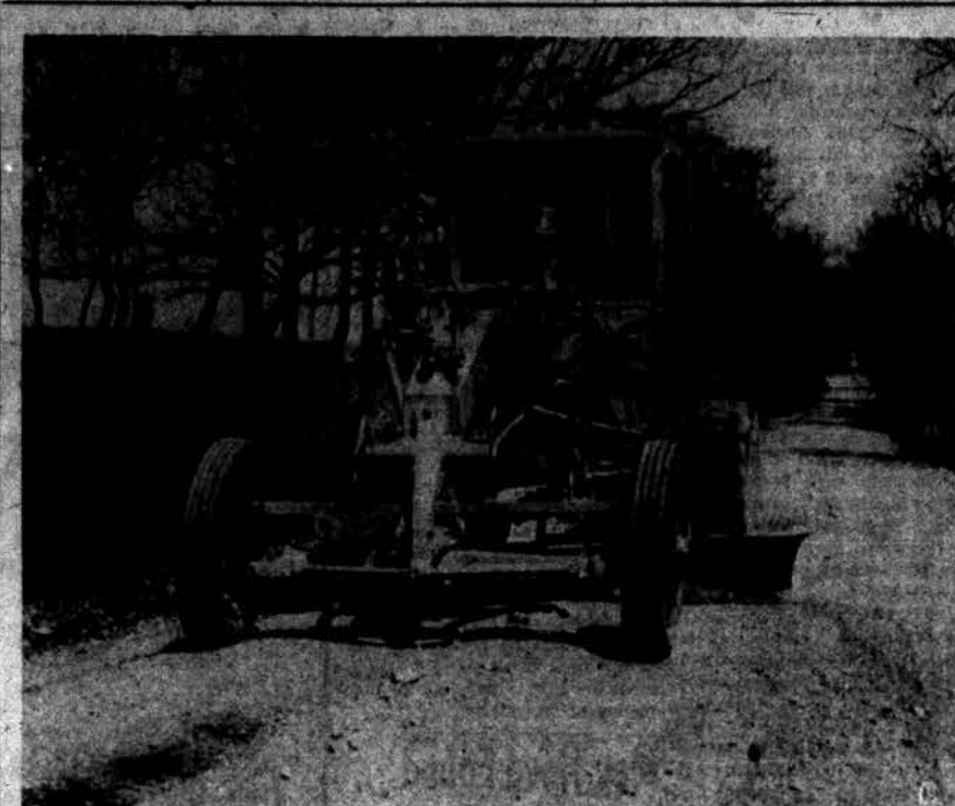
IT'S FIX-UP TIME — The Oakland County Road Commission is in the process of repairing roads throughout the county which were damaged by the ravages of a particularly hard winter. A typical sight in rural areas is the road grader leveling the gravel and filling deep chuck holes which have caused many a car spring to give under the strain this year. This machine was in operation on the Clarkston-Orion road.
