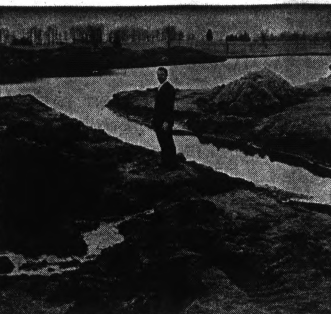
CHANGING COURSE — Club manager Lloyd Syron stands alongside some of the construction that is under way at the 10th hole of Pontiac Country Club. The changes are designed to alleviate the drainage problem in the area.
