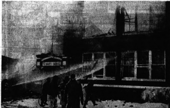
FIGHT SCHOOL BLAZE — Fire yesterday completely destroyed St. Mary's Elementary School in Gaylord despite efforts of Gaylord, Gaylord and Michigan Conservation Department firemen to save the two-story brick and wood building. The 309 pupils
