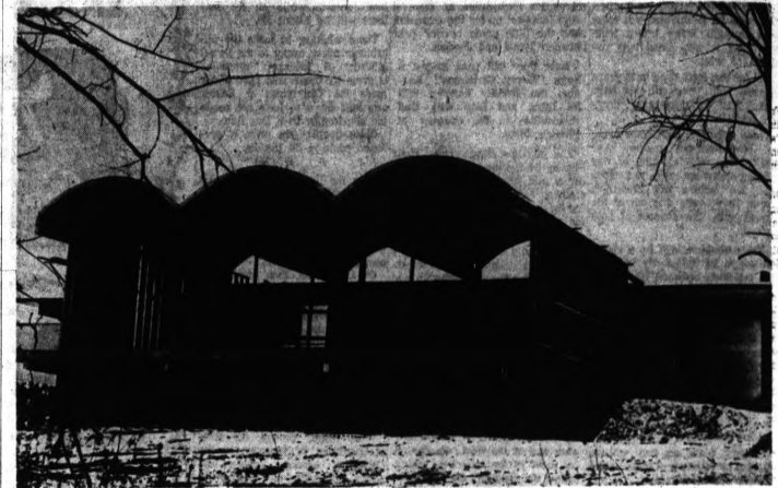
LIBRARY UNDER CONSTRUCTION — Work on the new $100,000 West Bloomfield Township public library will continue through the winter months with completion scheduled in February. Shown is the rear of the building with its canopied multipurpose room. Designed by the Birmingham architectural firm of
