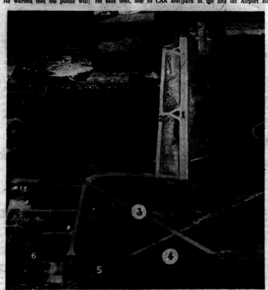
AIRPORT TODAY—Shown in this aerial photograph is the layout of Pontiac Municipal Airport as it looks today. You are looking west. The latest addition is the new 4,000-foot east-west runway (1) and the paralleling 6,000-foot taxi strip (2) which jogs down to connect with the north-south runway (4) and the two large hangers
