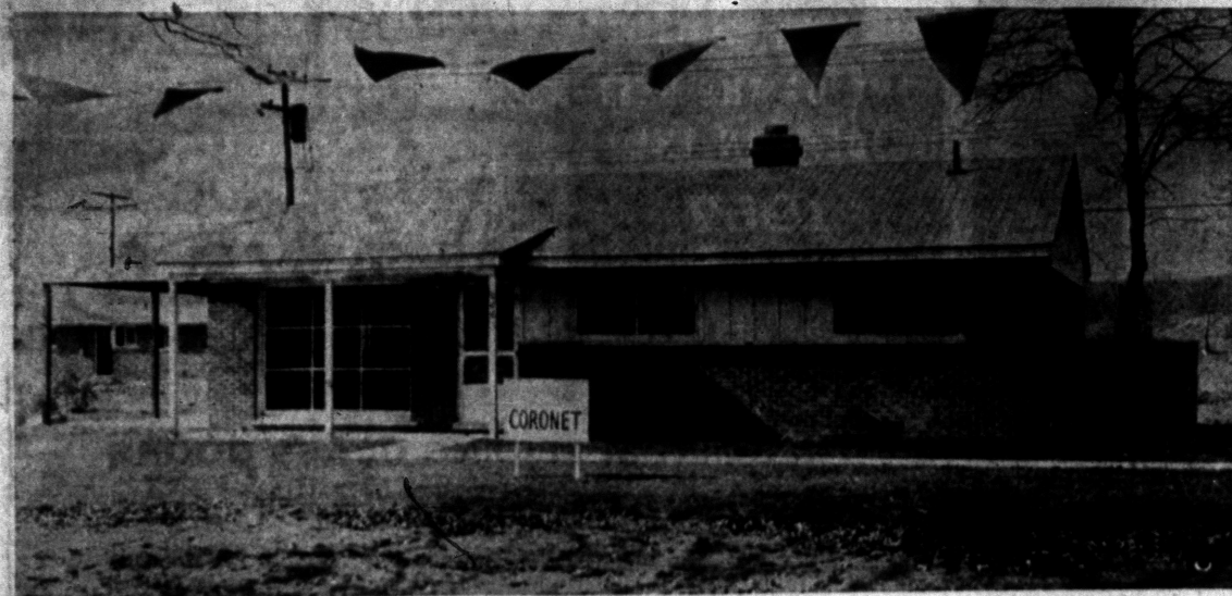
CORONET MODEL — Shown above is one of the two model homes in Mt. Royal subdivision. Located on 100x150 foot lots, the brick and siding homes are three-bedroom models. This model has one bathroom and a carport, while the other model has two
