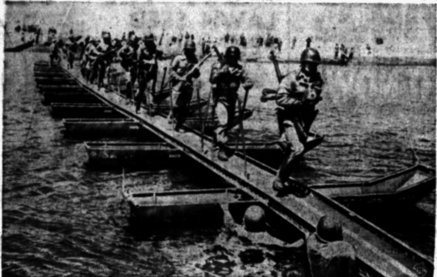
Combat Troops, carrying their weapons, race along the bridge's long span. Two maintenance men in the water keep a sharp eye on the condition of the bridge.
