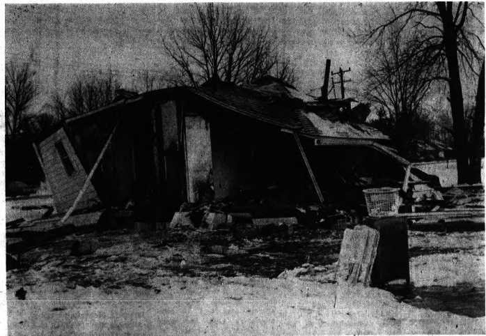
HOME EXPLODES — Mr. and Mrs. J. C. Reagan, 1713 Auburn, Avon Township, were vacationing in Florida when an explosion, reportedly caused by escaping gas, destroyed their one-story frame home at 3:20 a.m. today. The Avondale Fire Department stood by until 6:30 a.m. while gas burned in the basement. No one was hurt.
