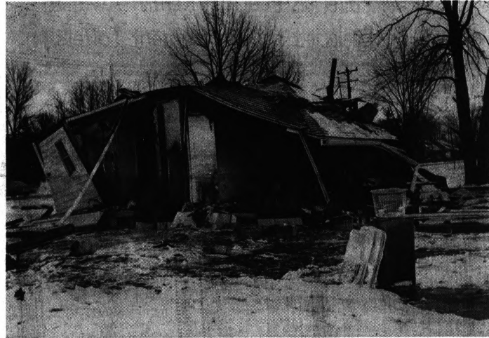
HOME EXPLODES — Mr. and Mrs. J. C. Reagan, 1713 Auburn, Avon Township, were vacationing in Florida when an explosion, reportedly caused by escaping gas, destroyed their one-story frame home at 3:20 a.m. today. The Avondale Fire Department stood by until 6:30 a.m. while gas burned in the basement. No one was hurt. Gas company officials said today no outside gas leaks had been detected and that a thorough check of the accident was being made.
