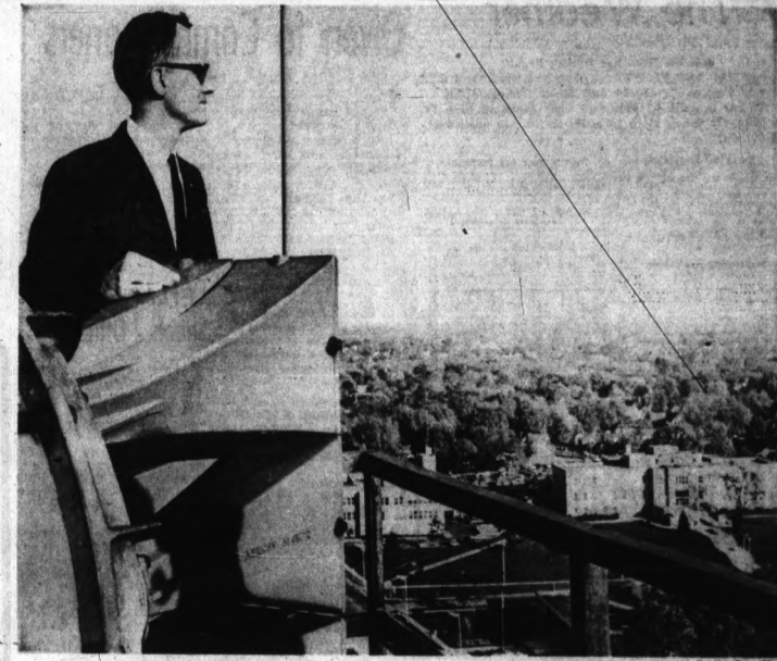
15 STORIES UP —The air raid siren atop the Pontiac State Bank Building, the city's highest office, is capable of throwing its warning din as far as 10 miles, according to Asst. City Manager Robert Stiller. Here he looks out over Pontiac and surrounding Oakland County from alongside the siren's mouthpiece. The siren is powered by a 18-horsepower gasoline engine and operated from a push-button behind the main desk in the Safety Building (partly shown beneath railing in picture). The $5,000 siren would be sounded as a warning to take cover from either enemy attack or tornado.
