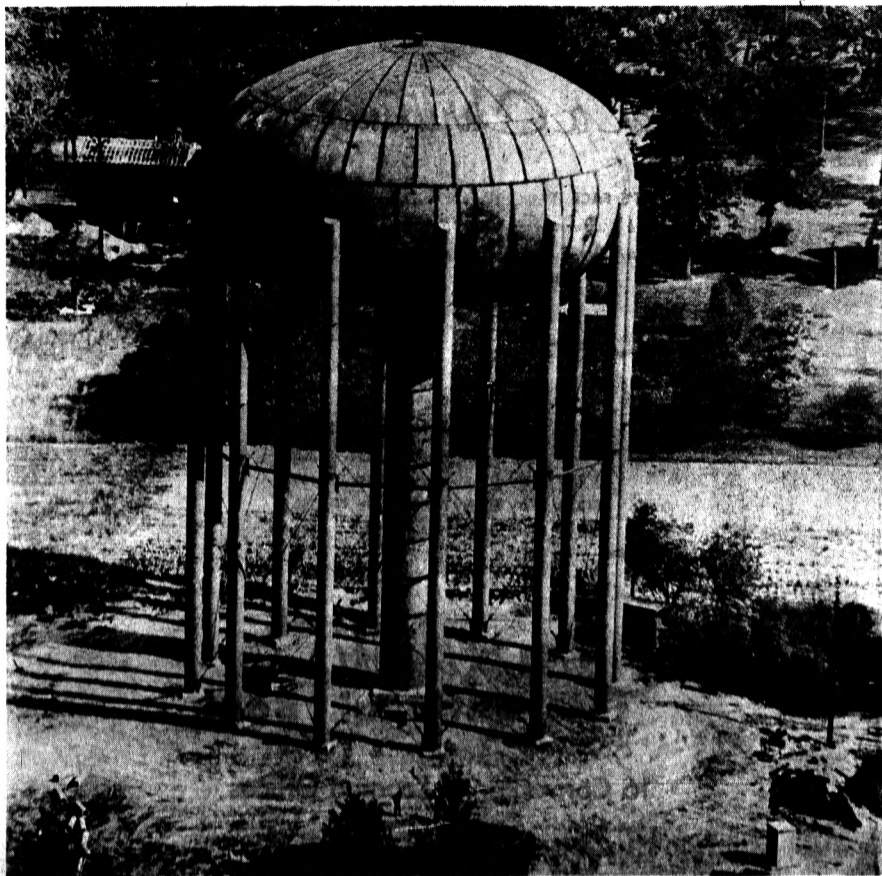
Elevated Tank At Shaddick And Mark With 1.5-Million-Gallon Capacity
