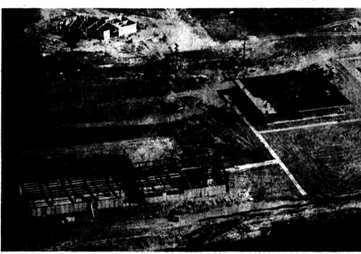
Water Department Buildings Under Construction
