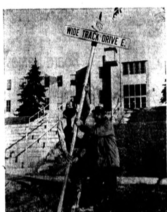
ERECT NEW SIGNS — A Wide Track Drive sign, one of 46 being erected on the newly completed road, is placed in front of City Hall by Department of Public Works employees Claude Day (left) and Robert Reynolds. Completion of the sign project is slated this afternoon. A dedication program is planned at 2 p. m. Friday at Wide Track and West Huron.
