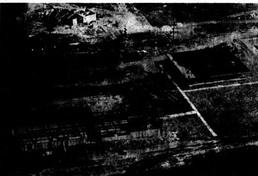
Water Department Buildings Under Construction
