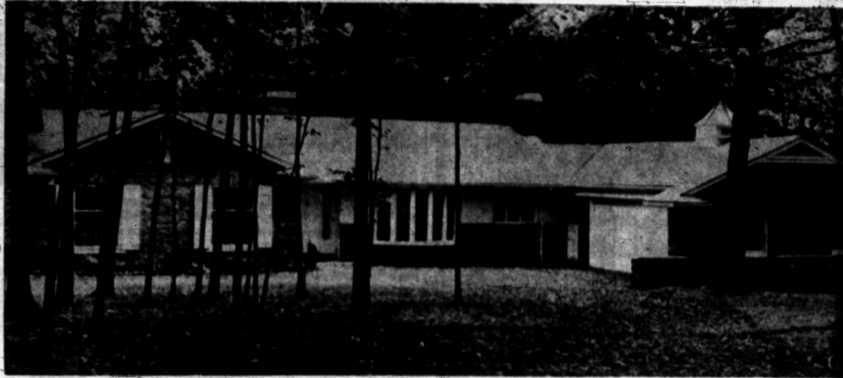
BESIDE A WATERFALL —In Forestbrook Hills, at the southwest corner of Twelve Mile and Inkster Roads, the George A. Duke Contracting Co. is building distinctive homes such as this Colonial
