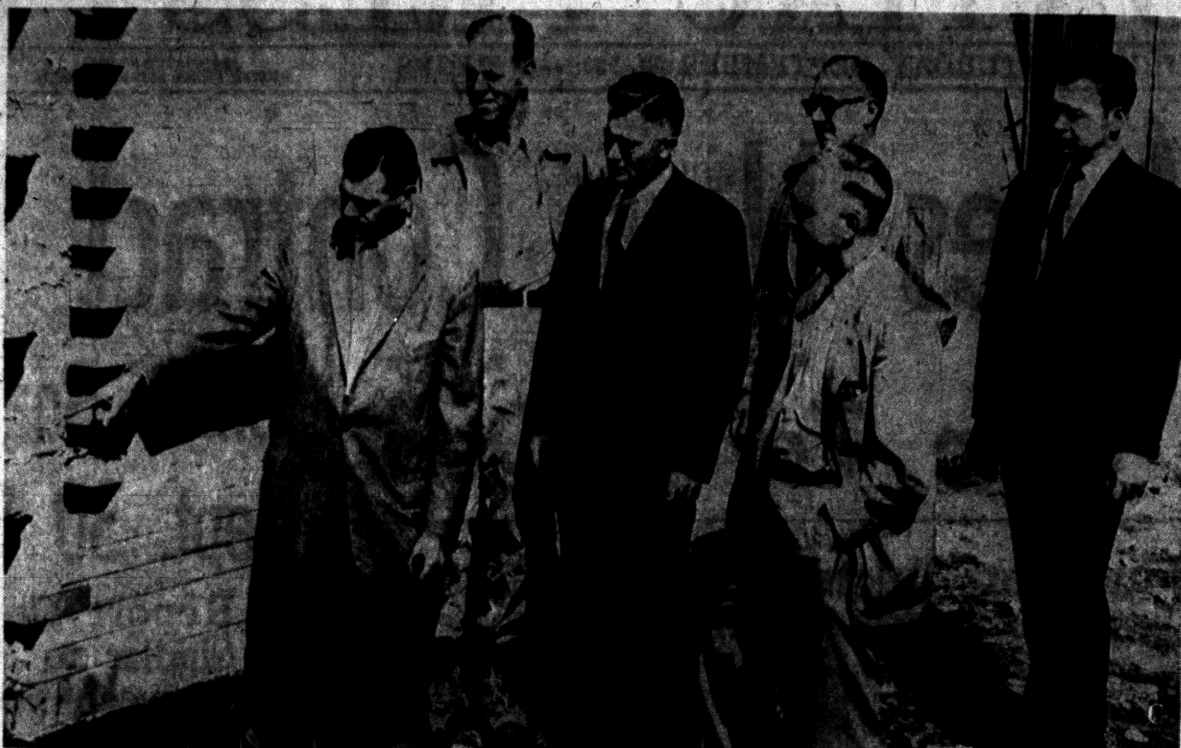
REVIEWING MSUO PROGRESS — At the monthly meeting yesterday of persons closely concerned with the erection of the Michigan State University Oakland building, Floyd Heineman, field supervisor for Swanson Associates, architects, points out progress on brickwork. Studying the building are, from left, Clarence Kremer, job superintendent for J. A. Fredman Construction Co., the general contractor; Theodore Simon, superintendent of buildings and grounds for MSU; Ray Westrick, secretary-treasurer of J. A. Fredman Co.; Donald O. Ross, supervising architect for Swanson Associates; and George Karas, supervising engineer for MSUO.
