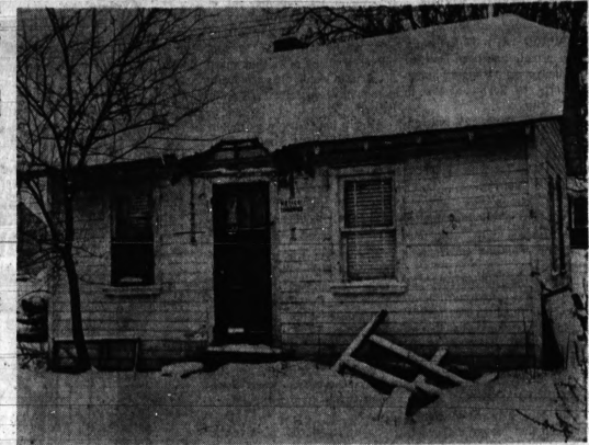
CONDEMNED — Snow covers the rubbish and debris in the yard around this back-lot house at 113 W. Colgate. A "condemned" notice has already been posted on this vacant structure on Pontiac's northwest side.
