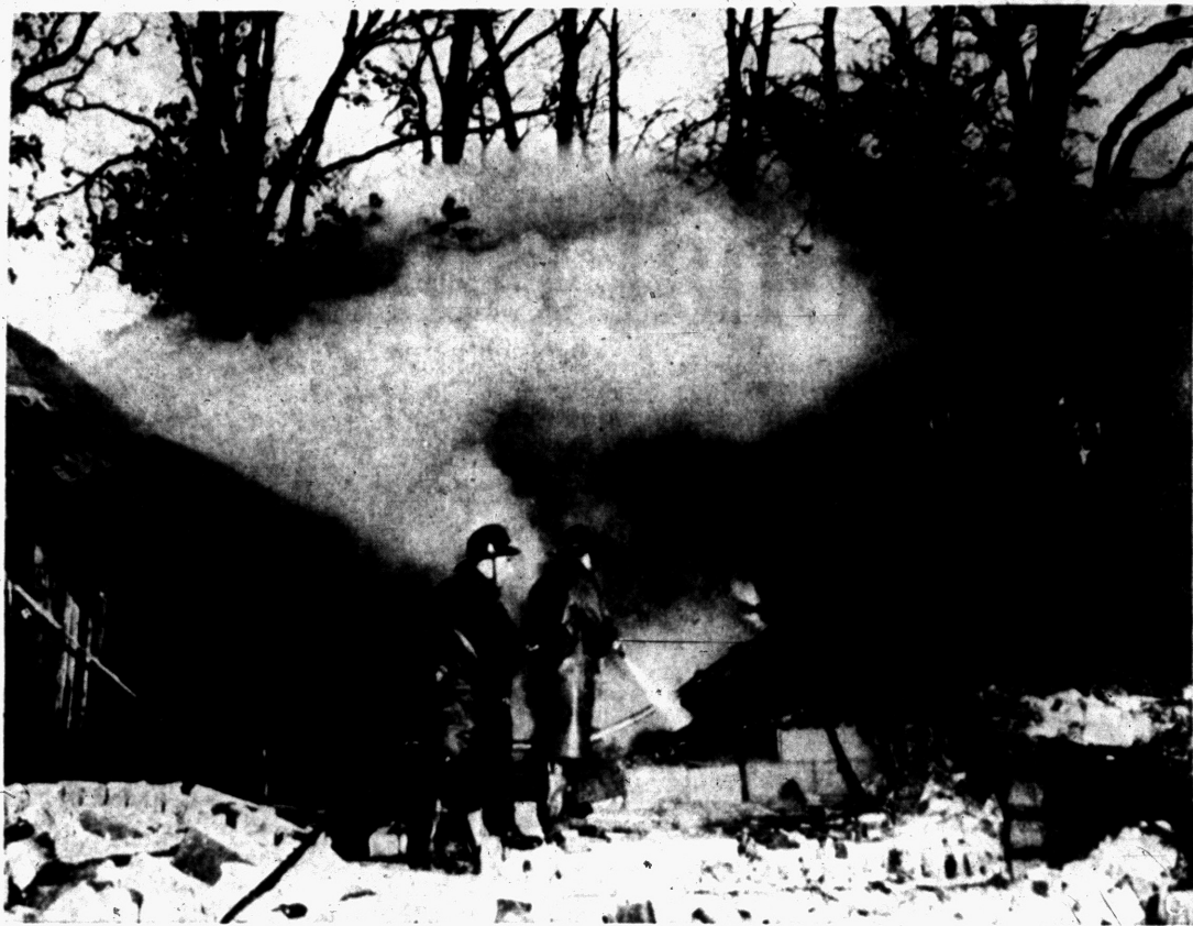
WHITE LAKE TOWNSHIP FIRE —Three firemen were injured in this blaze Sunday afternoon when combustion in the hay-filled three car garage blasted the roof in and the walls out. The fire, at
