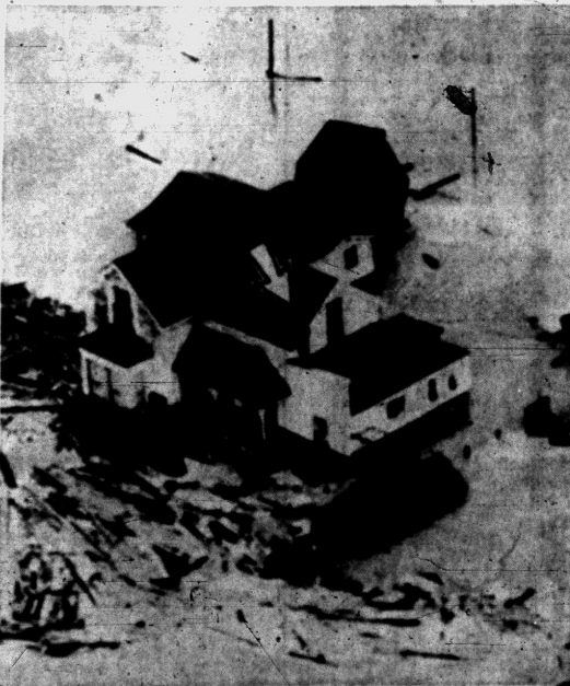
FLOODS HIT WEST COAST — Late in December floods described as worst in West Coast history hit three states, causing loss of life and extensive property damage. Above, a farmer stands atop his flood-marooned home south of Eureka, Calif.
