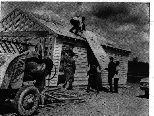
LEARN BY DOING — Getting practical experience are Oxford High School carpentry students as they build a garage for the storage of maintenance equipment. Guiding the project was Elmer Ball, the carpentry
