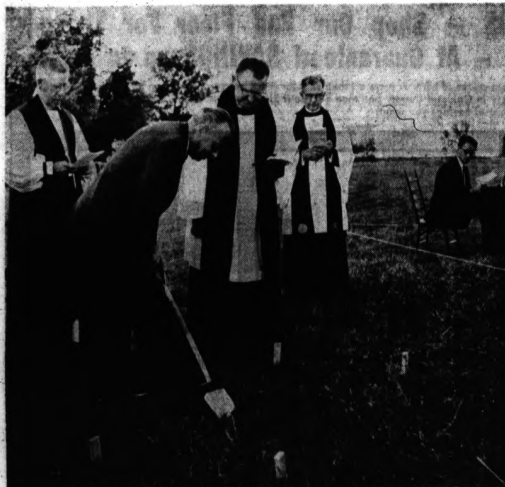
NEW CHURCH — John DeLind wielded the shovel yesterday at groundbreaking ceremonies for the new building that will house the Episcopal Church of the Resurrection near Clarkston. Located on a four-acre site at Clarkston-Orion and Perry Lake Roads, the church is scheduled for completion early next year. Participating in the ceremony (from
