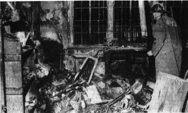
BLAST RUINS AT PRISON — A Blackman Township fireman checks the smoldering ruins of the arsenal at the State Prison of Southern Michigan which blew up last night killing two prison guards. The explosion also knocked out electric
