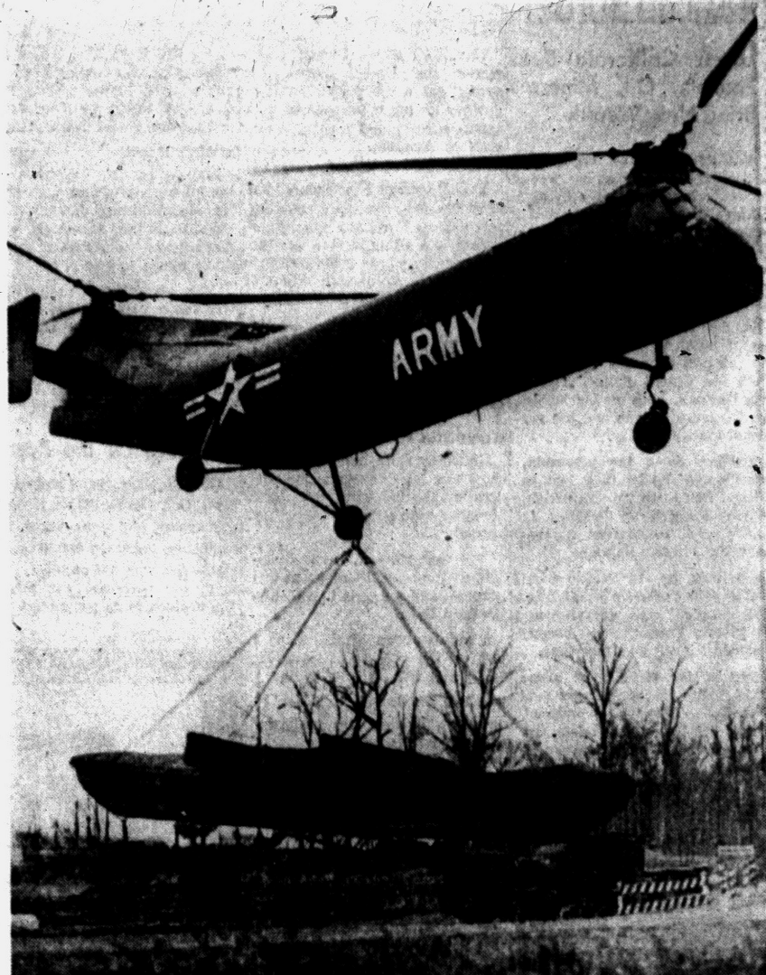
BRIDGE IN FLIGHT — A hovering helicopter once again proves itself almost as versatile as an Army jeep as it lifts a section of bridge weighing 2,900 pounds during a test operation at the Fort Belvoir, Va., Corps of Engineers Research and
