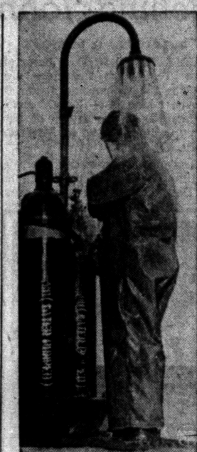
HOT SHOWER — Included in newest Army methods is this "hot" shower designed to wash decontamination from soldiers exposed to radioactivity in training, or warfare. Its most frequent use comes at guided missile sites, where men come in contact with liquid fuels for the missiles.
