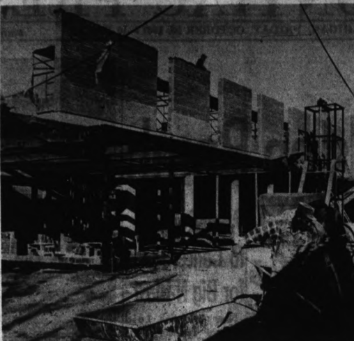
FIRE STATION GROWING — Pontiac's new central fire station is entering final stages of construction on East Pike Street across from the Public Safety Building. The entrance ramp has been poured and work is about finished on walls for the kitchen and dining room sections.
