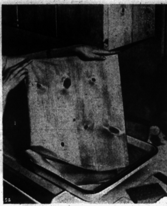
PLASTIC FILM dipped in warm water makes it easy to transform plain kitchen cabinets to knotty pine paneling.
