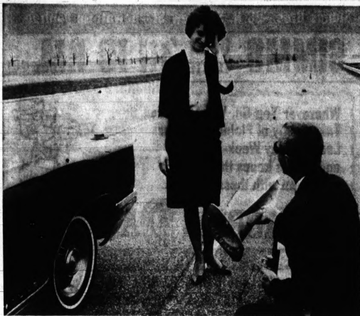
CONE CRUSHER —A smashed highway marker dismays Jo Ann Cain, but it helps General Motors design a safer car. A typist, Jo Ann is one of the 25 GM Proving Grounds volunteers who test-drive experimental combinations of automobile controls to find the one best suited for the average driver.
