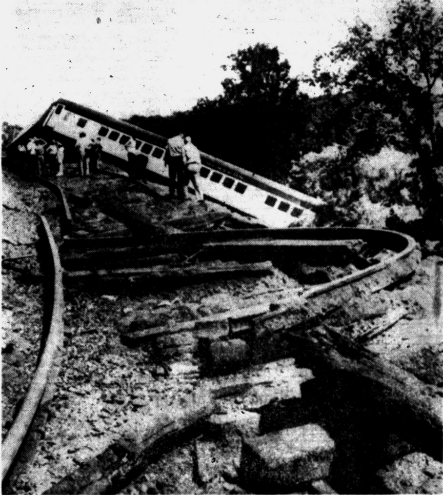
ACCIDENT SITE — A twisted rail speaks a silent epitaph as workmen and officials mill around the scene of yesterday's train derailment in Wisconsin in which at least 100 persons were injured. Seven cars of the speeding train left the tracks and three slid halfway down a 100-foot embankment before they were stopped by a clump of trees. It was thought that heat might have snapped a rail, causing the accident.
