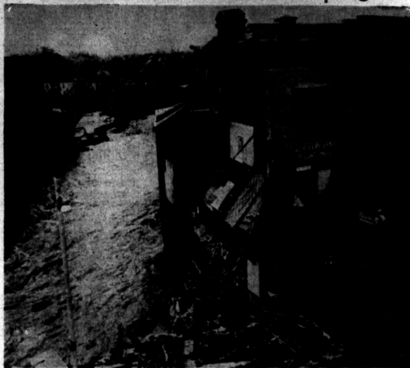
WATER ON A RAMPAGE —The flood-swollen Norwalk River is shown above as it sweeps past debris of a destroyed Norwalk, Conn., waterfront building yesterday as rain continued to lash southern New England.
