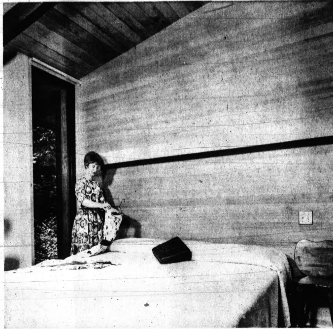
PANELED HEADBOARD - Here's a good bedroom decorating idea - use an elegantly paneled wall in place of a headboard. Horizontally installed west coast hemlock panel boards stretch the room's width and give a silky smooth look. A lighting soffit, made from a single matching board, creates accent and provides good reading light.
