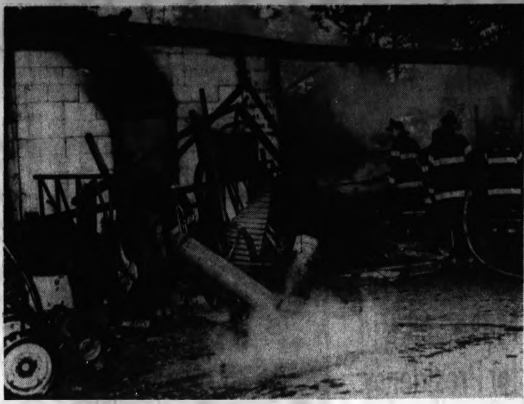
BUILDING DESTROYED—Tony's Welding Shop, 355 E. Walton, Pontiac Township, was destroyed Saturday in this fire which took the lives of two men. The owner of the shop, Anthony Adamo, was welding a hitch on a car when sparks ignited the blaze. Adamo, alone in the shop at the time the fire started, escaped unharmed.
