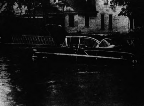
PONTIAC CREEK FLOOD—Automobiles in the Pontiac Press parking lot just north of West Huron Street in downtown Pontiac stand in head-high water after Pontiac Creek overflowed its banks during yesterday's vicious thunderstorm. Flooding rainwater overflowed, the curb in many spots in the downtown areas.
