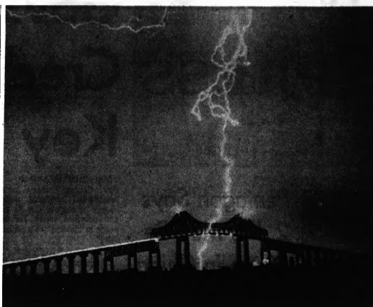
EMBROIDERED SKY —The 150-foot high Sky Way Bridge across Tampa Bay in St. Petersburg, Fla., is etched against the stormy night sky by bolts of lightning. This area has more electrical storms than anywhere in the country.
