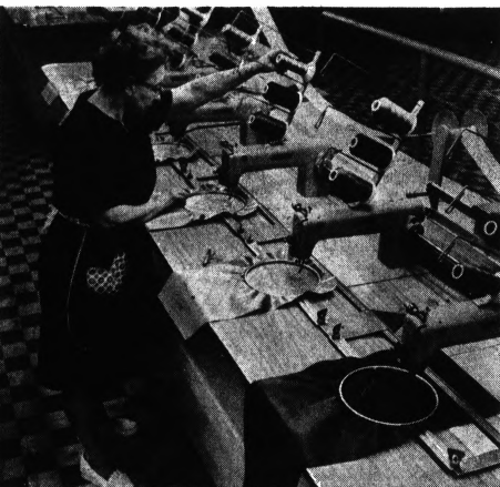
Intricate embroidered patterns are constantly checked for loft, dimension, contour and design. As the pattern is completed, the machine will automatically stop.
