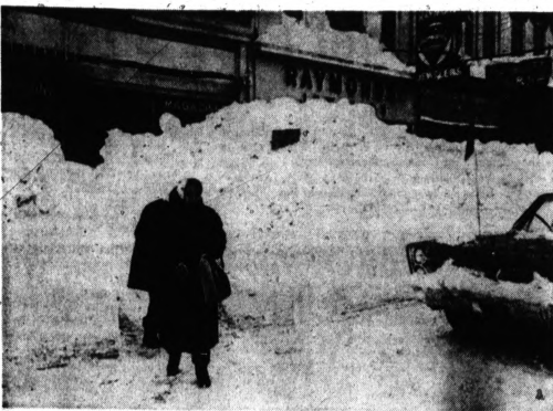
CHANNEL TO BUSINESS —This is Bridge Street in Oswego, N.Y., the principal thoroughfare when it reopened for business after recovering from the blizzard-inflicted
