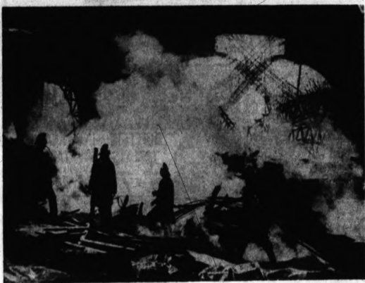
FLAMES AT U.S. EMBASSY—Amid an impressive background of twisted steel arches and smoke, Mexican firemen fight to subdue the rampaging fire which destroyed the eastern wing of the U.S. Embassy building under
