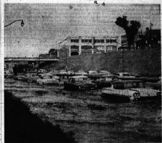
AQUACADE ON XWAY — Automobiles crawl through water that backed up on the Edsel Ford Expressway in Detroit Friday after a freak storm flooded storm sewers on the west-bound lane.
