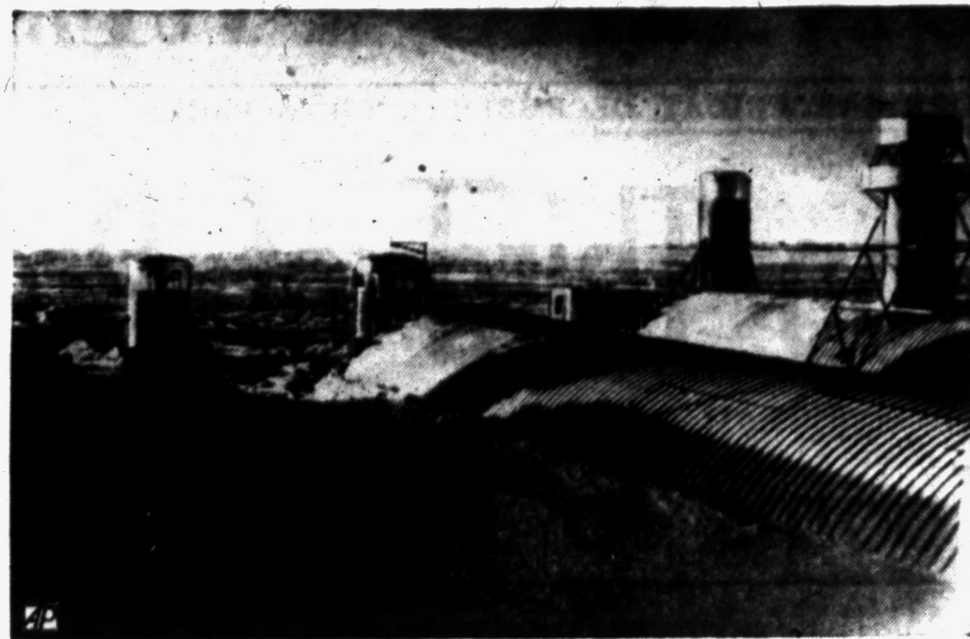
SINKING BASE BUILT IN GREENLAND —The Army released this photograph in Washington this week showing a new arctic military installation designed to sink slowly into the soft snow of the Greenland polar icecap. Buildings in foreground are steel tubes 18 feet in diameter. Vertical entrance towers are used. As the buildings sink, new sections are added to the towers to keep them above ice. Buildings are designed to sink several feet a year. Inside are quarters for several score Air Force men operating the weather observation station.
