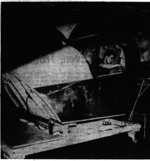
NEW ESCAPE COCKPIT — Mechanics William Hester (inside) and C. F. Baldrige work on a new jet plane escape cockpit at McDonnell Aircraft Corp. in St. Louis. It is
