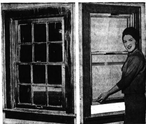
Before Old window is unsightly, hard to wash, rattles, lets in drafts and dirt, has rotted sills and frames.
