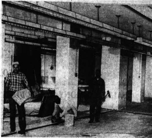
FEDERAL FACELIFTING—The Federal Building at East Huron and Perry streets has been undergoing a gradual facelift since the main post office moved to new quarters several years ago. Most of the old post office area has already been remodeled to house federal agencies and the entire project should be finished by this fall. Shown here (from left) are Earl Harkin of Dearborn, Randall Gillette of Inkster and Tom Stokes, 330 First St., working on final stages of the vast modernization project.
