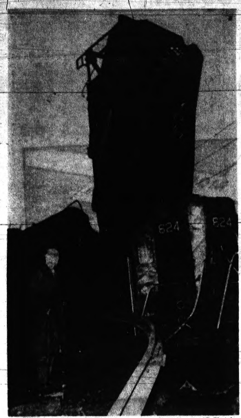
RAIL STOCK GOES UP — Flatcar of a Reading Railroad freight train stands upright after the 10-car three-engine train hit an open switch and derailed in Edison, N.J. Four trainmen were hurt in the crash.
