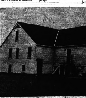
MEMBERS BUILD ADDITION — Except for the basement, the new Sunday School addition to the Gingsville Baptist Church was built by the members. It is the wing at the left in this picture
